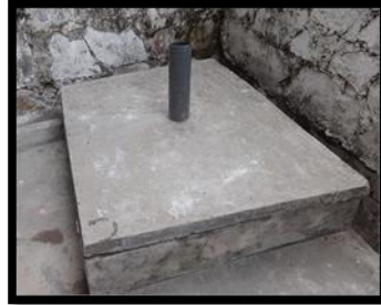
Concrete Sharp Pit
